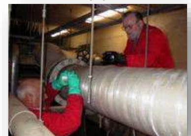
Quickly stop leaking pipe work & provide further integrity
